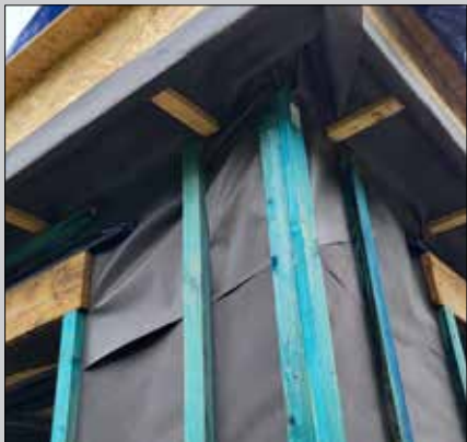
Leave membrane loose at the top as this will extend over the OSB fascia later in the build as shown in the example above.
