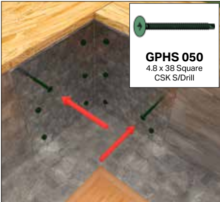
Secure internal cleat using GPHS050, 6 per side and repeat for all corner joints.
