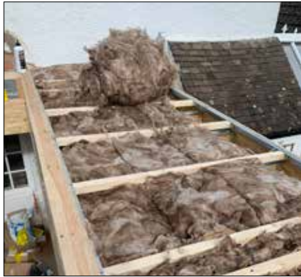
Before fitting the OSB decking fill the gaps between the firrings with insulation.
