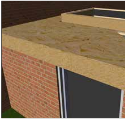
Continue around, gluing and placing until a full section is complete. Note: Boards are oversized at drip edge to be cut back to suit drip detail being fitted.
