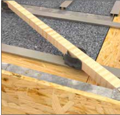
Continue placing and securing Pitchlocks inline and in conjunction with the location plan, placing them no further than 1m apart. Once completed, place firring in position.
